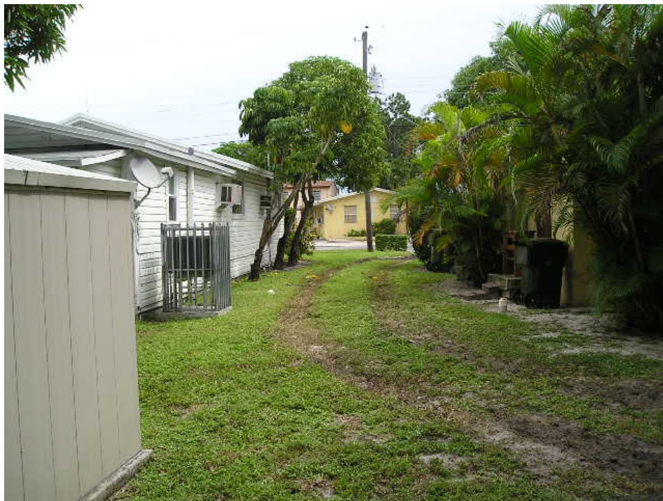
2. VIEW EASTERLY ALONG THE CENTER OF THE SUBJECT PROPERTY ( showing portion of shed that may encroach onto subject property ) TOWARD SW 5 AVENUE
